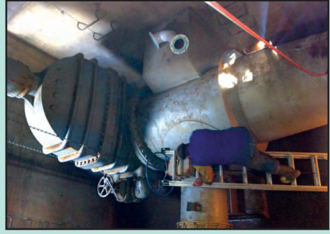
Brian Taylor, Pipeline Forman for Casitas climbs down into Casitas' three-way structure.
